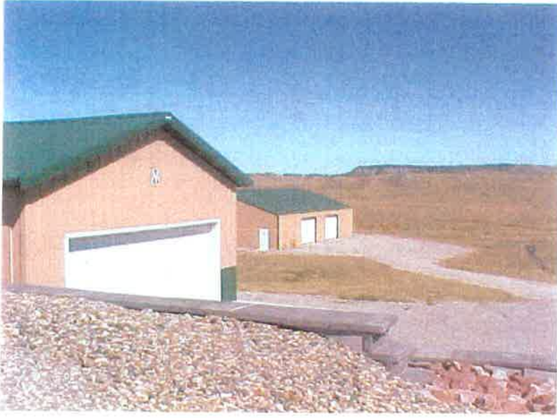
Garage and the shop/barn
