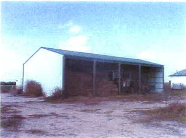
OPEN FACED MACHINE SHED: Built 2005, metal/pole barn construction.
