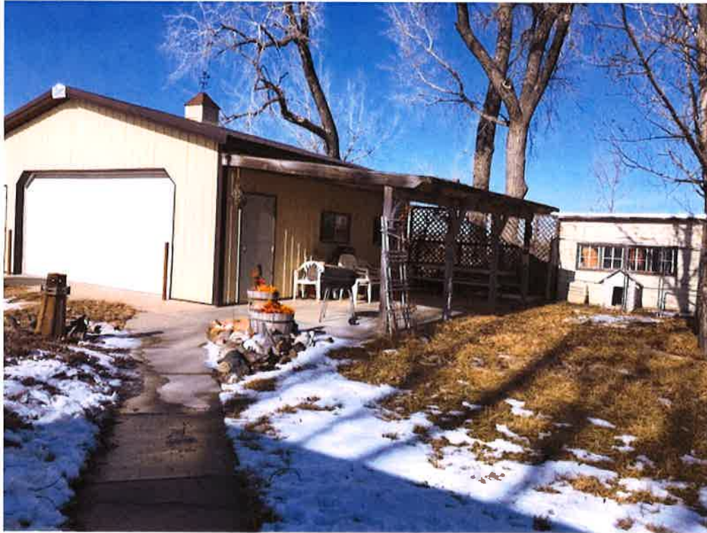
The 24 X 30 Cleary shop/garage building has an attached covered patio perfect for summer cookouts.
